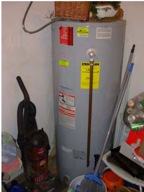
9. DHW tank serving the community facility
