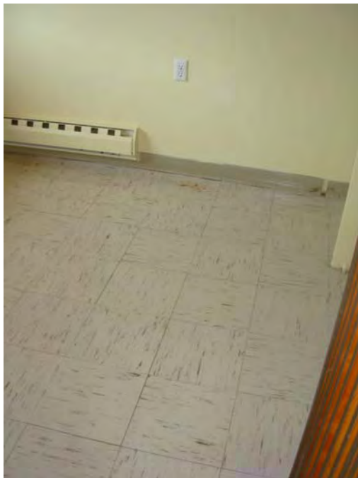
11. Vinyl tile flooring seam separation, marking Gladys Green Apartments • Capital Needs Assessment • © On-Site Insight
