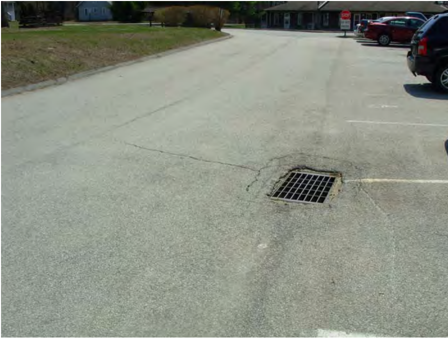
1. Spot cracking of parking surfaces
