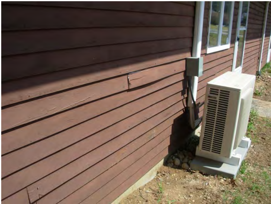
5. Wood siding deterioration and damage
