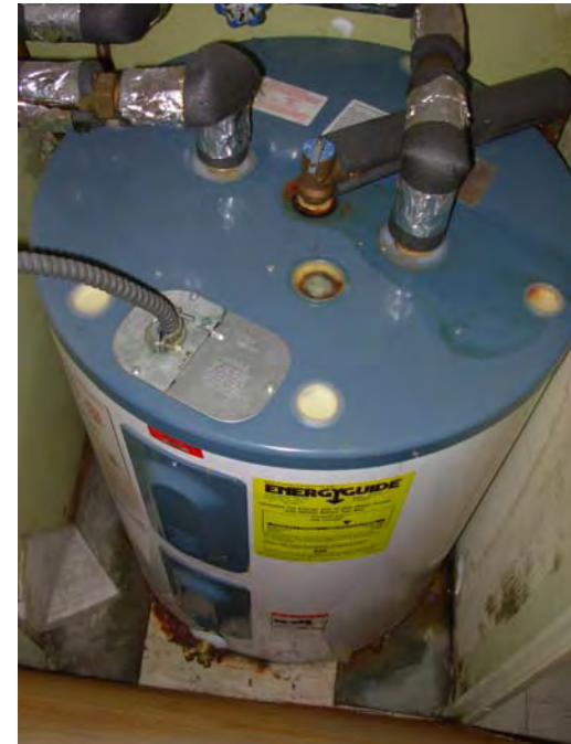
16. Typical DHW tank serving unit hot water needs
